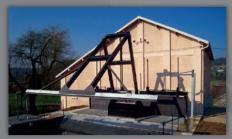
Fixed trash rack cleaner with channel discharge (fish friendly)
